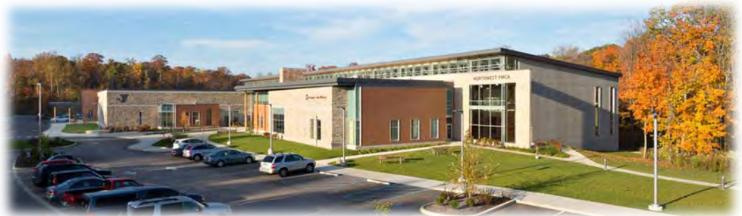
This image shows a local athletic facility combined with office space. The building pictured incorporates several types of materials that are encouraged by the City of Darien, which are natural and precast stone, architectural precast panels, and glass.
